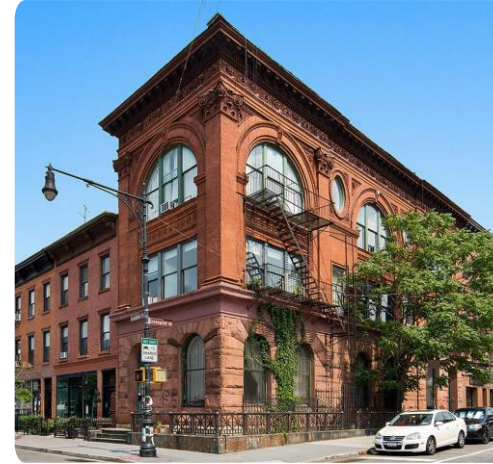
Mechanics and Traders Bank of Brooklyn Building GREENPOINT 1985
